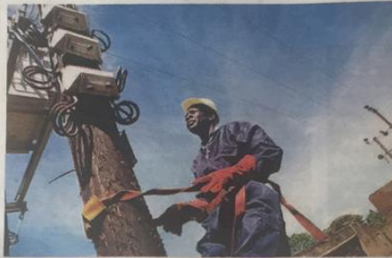
An engineer connecting electricity
